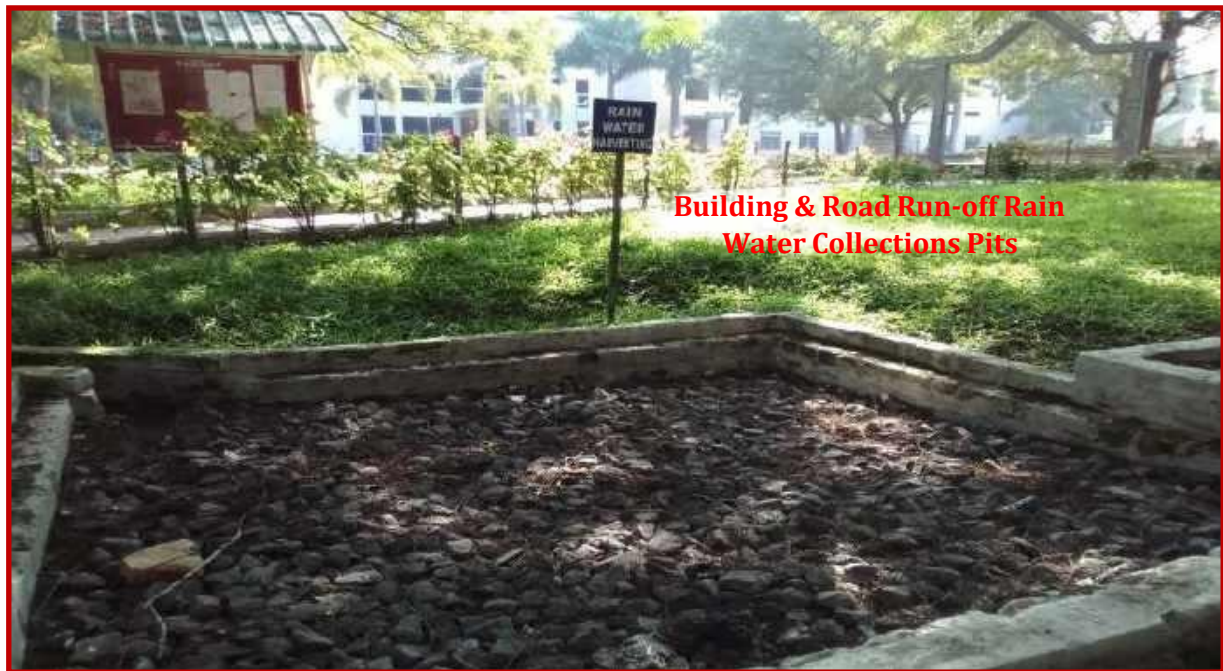
Fig.4: Rain Water Harvesting (RWH) system implemented in the College
