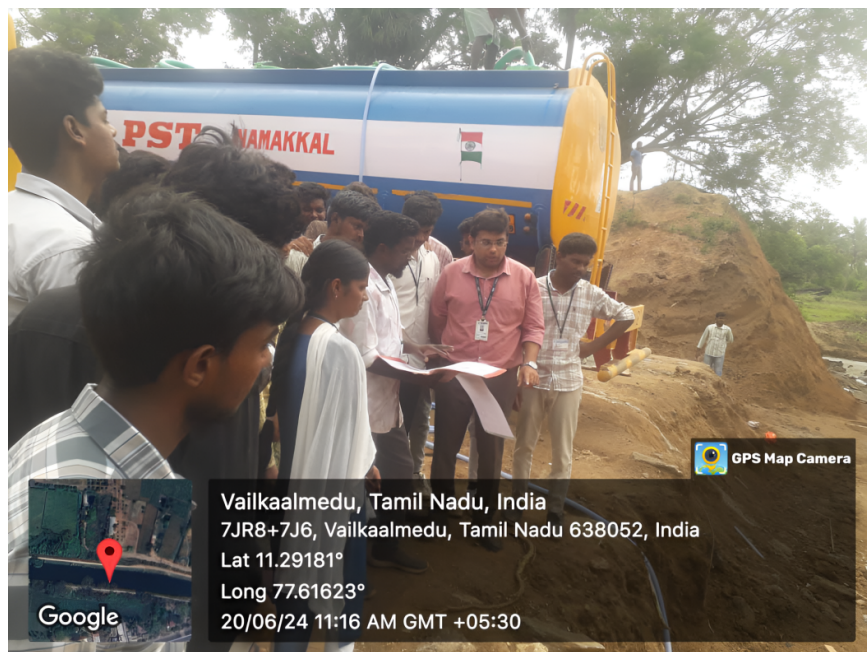
IV year Civil Engineering students at drain culvert site on 20.06.2024
