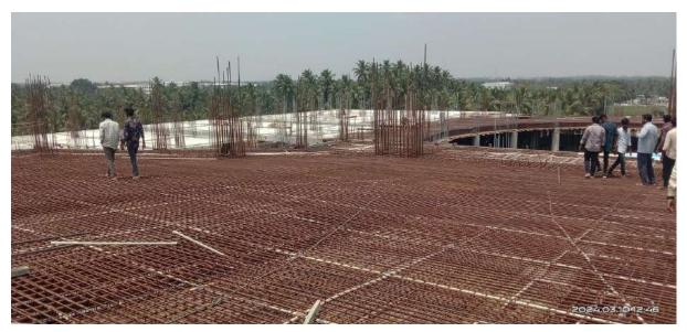
Both one way and two way slabs were reinforced on the day of visit. Students were able to differentiate tension and compression reinforcement. The conditions which demand extra reinforcement were also discussed.
