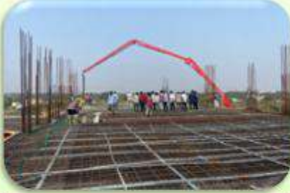
Site Visit during Boom Pumping Concrete
